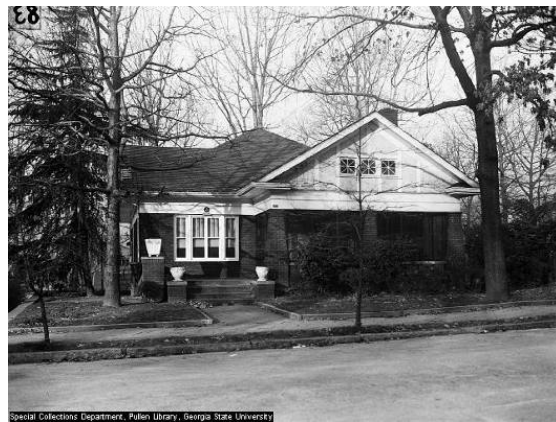
Special Collections Department, Pullen Library, Georgia State University
